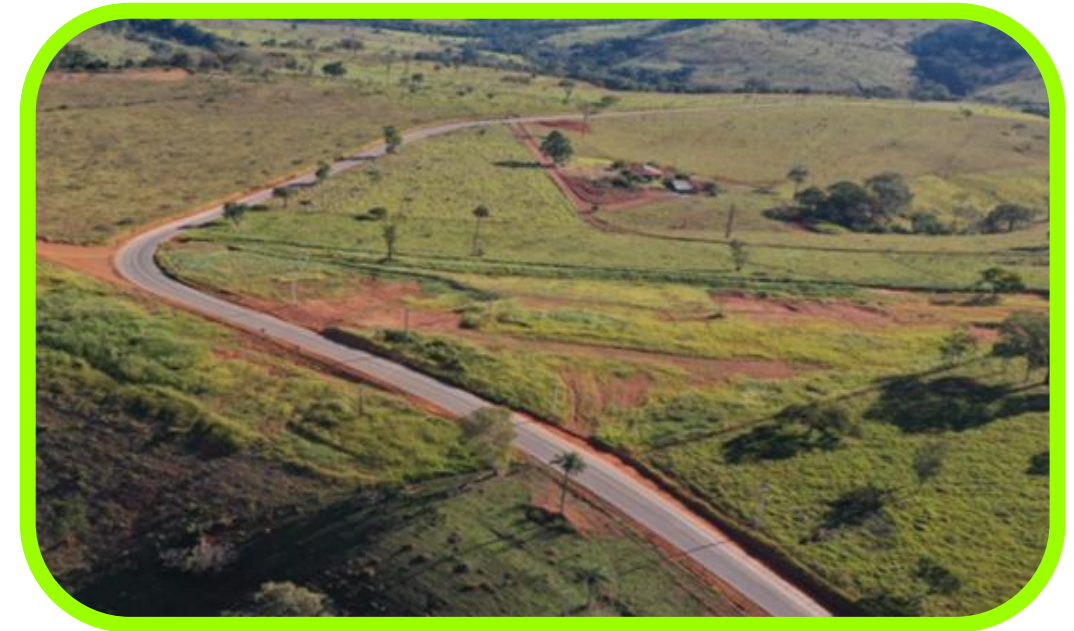
Currently paved area.
