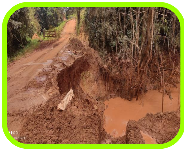
Before- Section with potholes and inefficient lateral drainage and boggy areas.
