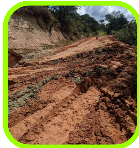
Before- Section with potholes and inefficient lateral drainage and boggy areas.
