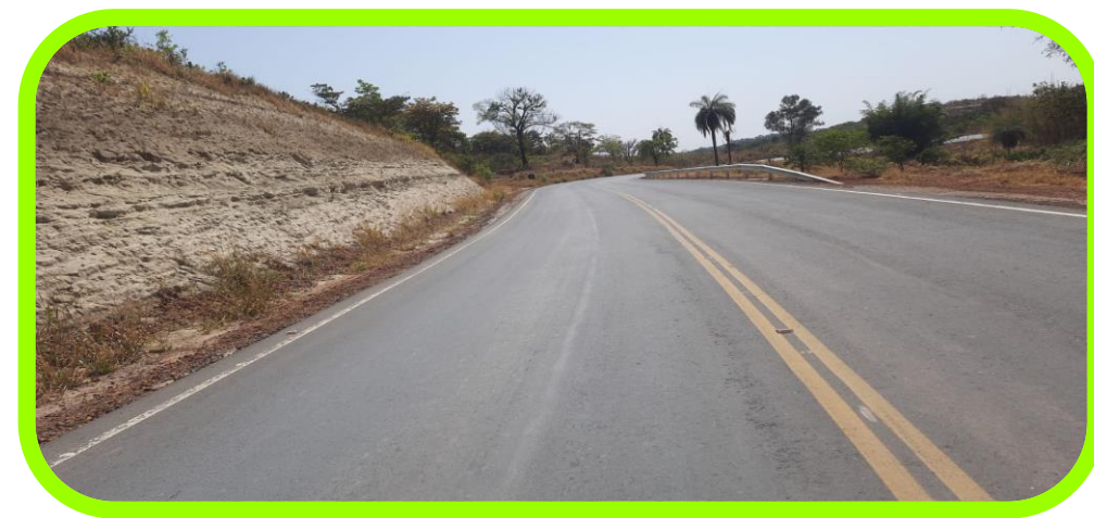
After – paved road
